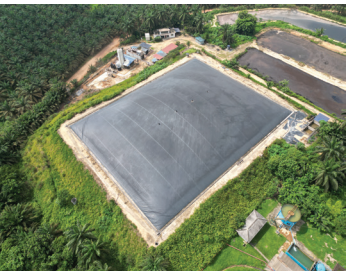
GLT Global Resources 1MW Biogas Power Plant
