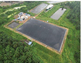
GLT Climate 2MW Biogas Power Plant
